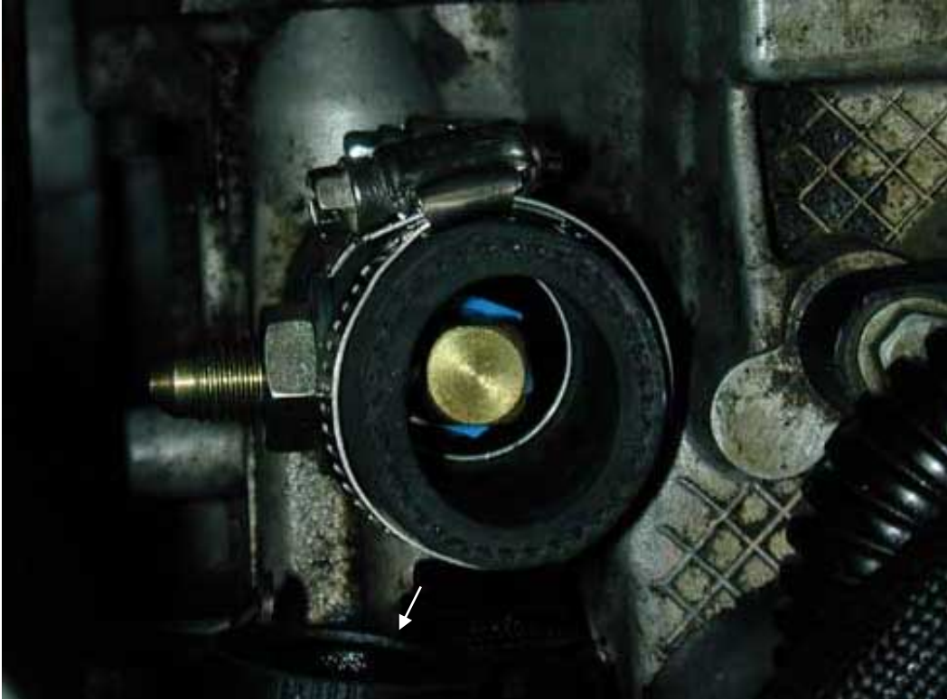
Photo 9.4. Oil return assembly installed with loose clamps.
