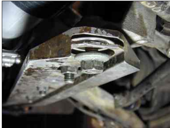
Photo 18.0. Nut flush with stud for stud removal.
