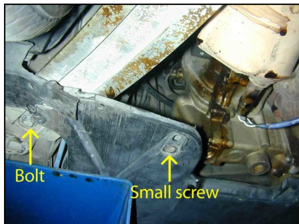
Photo 4.1 Support strut fasteners.
