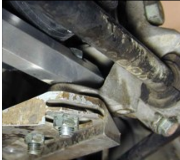
Photo 18.1. Cross Brace installed.
