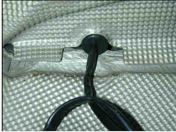
Photo 11.8. Harness grommet installed.
