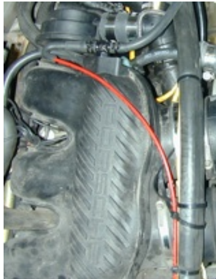
Photo 19.0. Boost Gauge vacuum line routing.
